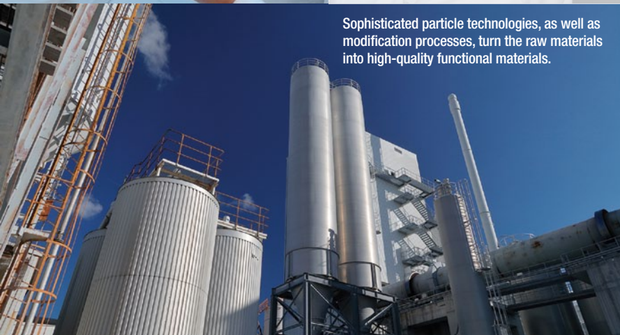
Dorfner supports e.g. the paint & coatings industry with solid application know-how.
